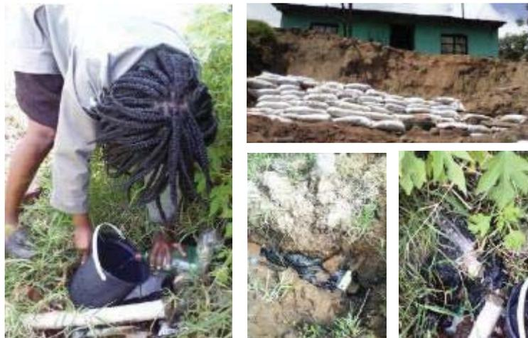
**Figure 51: Images showing the damage to the infrastructure in Ezimbokodweni, as well as one of the Wise Wayz Water Care volunteers measuring the outflow from the leaking pipe (right). The images below left show the damaged pipe.**
